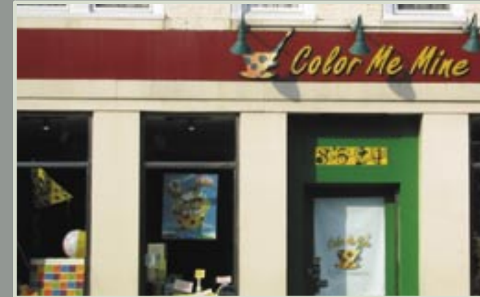
Letters painted on the wall, externally illuminated.
