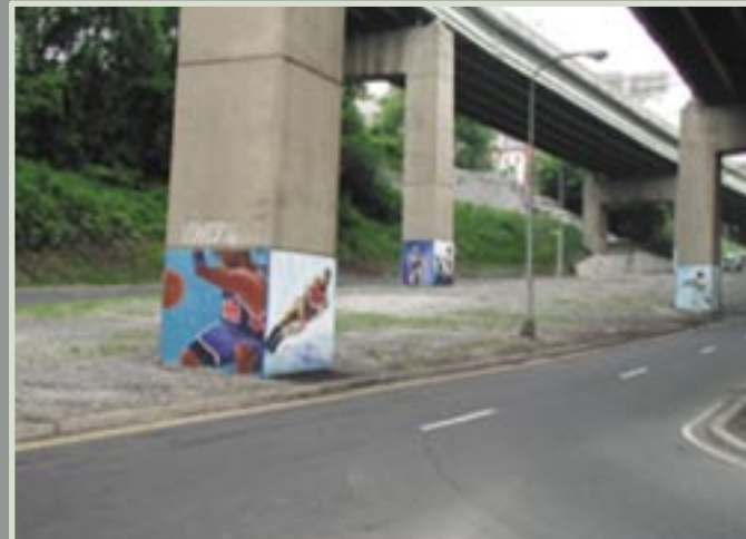
Abutments under Rte 1 present an opportunity for public art, and the paved ground can be landscaped with ground cover and flowers.
